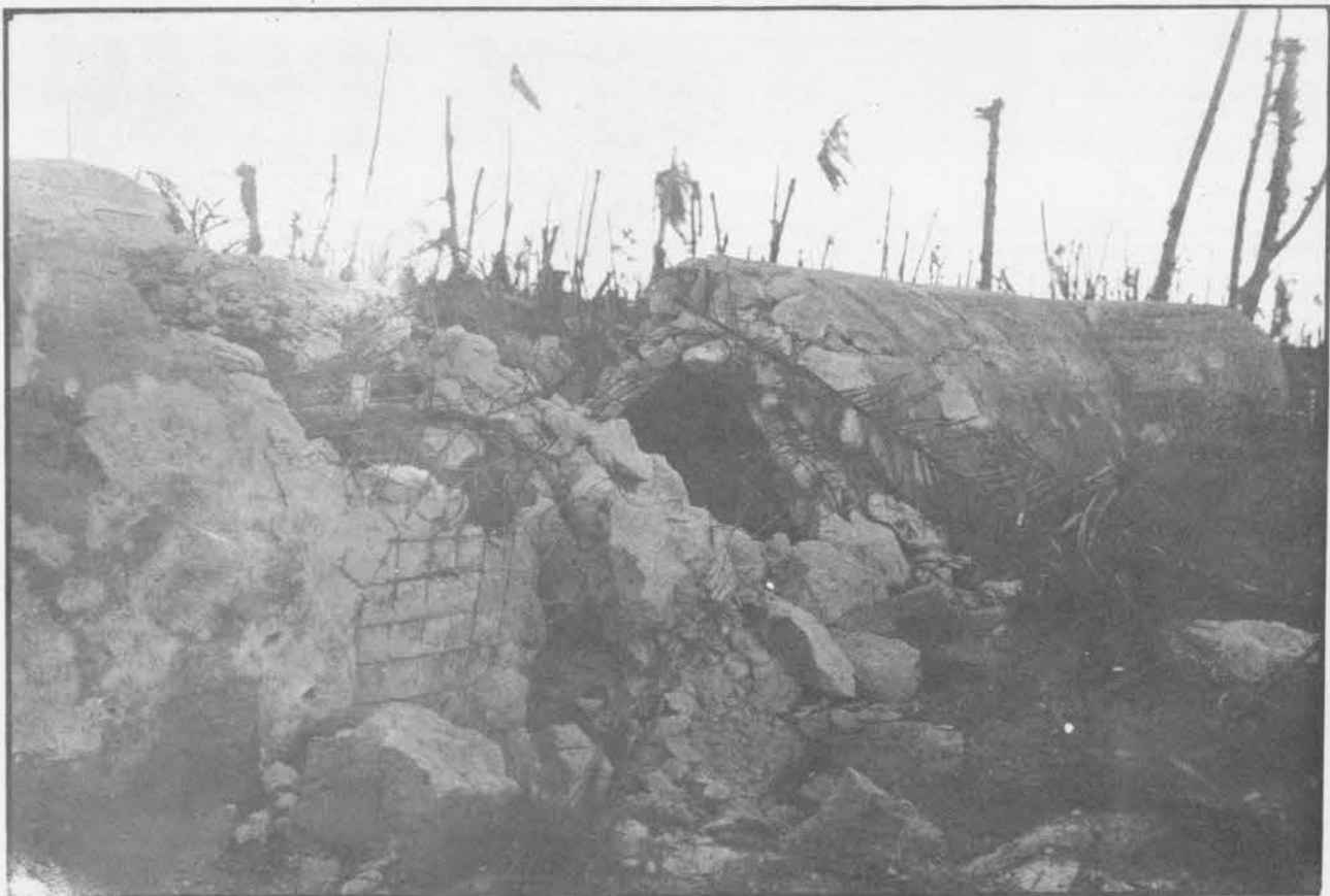
EFFECT OF GUNFIRE AND BOMBARDMENT OF AIR RAID SHELTER, EBeye
