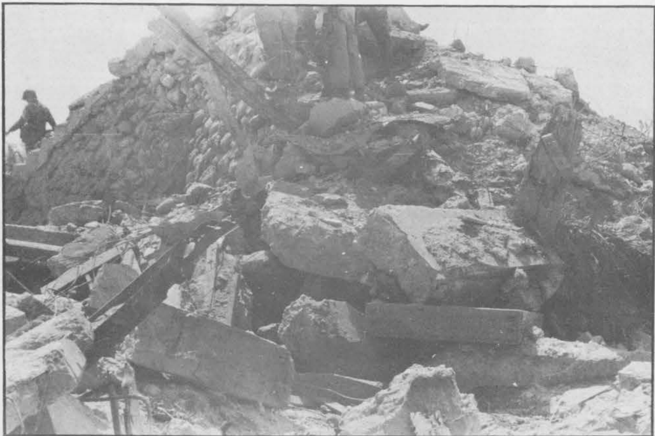
EFFECT OF BOMBARDMENT OF 5" AMMO MAGAZINE, KWAJALEIN
