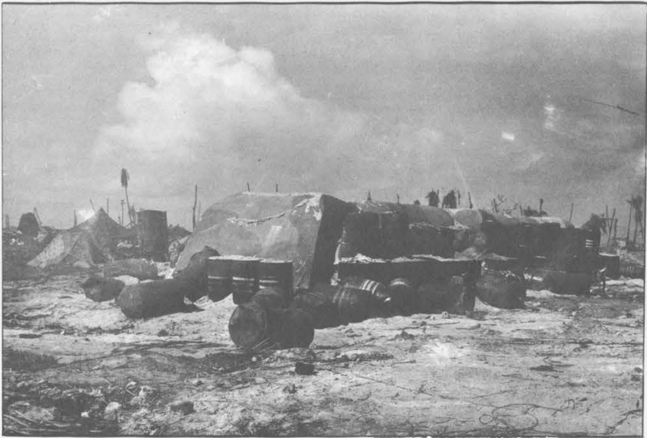
METHOD OF REINFORCING AIR-RAID SHELTER WITH USE OF SAND FILLED EMPTY GASOLINE DRUMS, ROI
